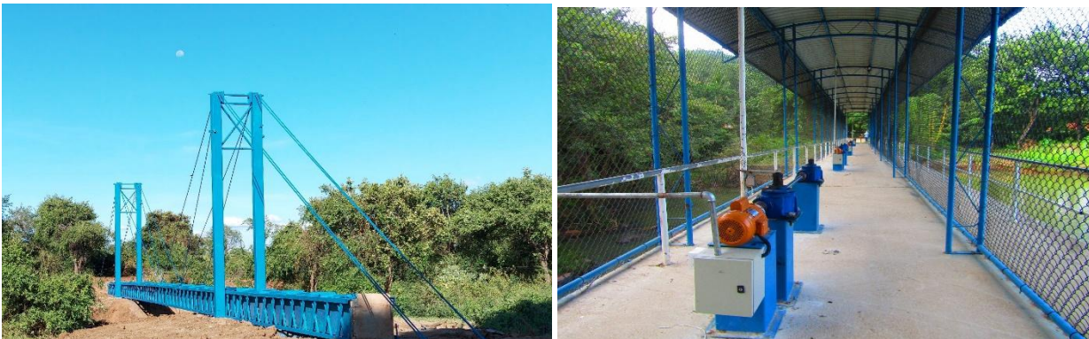
Dewliya wewa suspension fiberglass aqueduct on GI structure and electromechanical gates and shelter at Kumbukkana anicut
